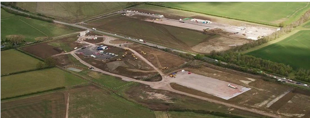
Ariel view of the A41 compound and temporary roundabout.
